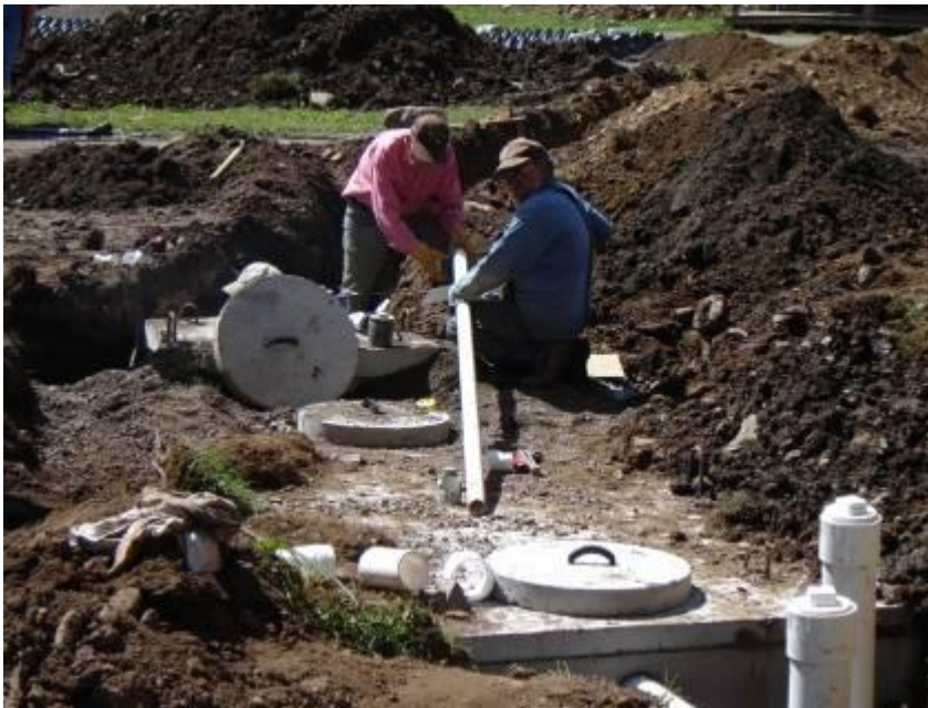
Figure 9. The Lodge's Septic Tank Installation in 2007 (Source: Conejos County Land Use office)
